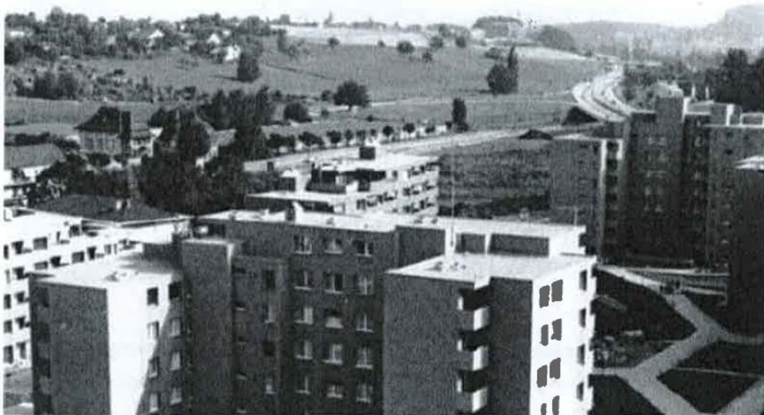
Figure 29: The settlement Paradies just after the construction phase (1972). The settlement consists of the five buildings.
